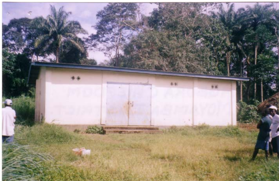
Photograph 5: Detention site at Magbenka, Moyamba District
