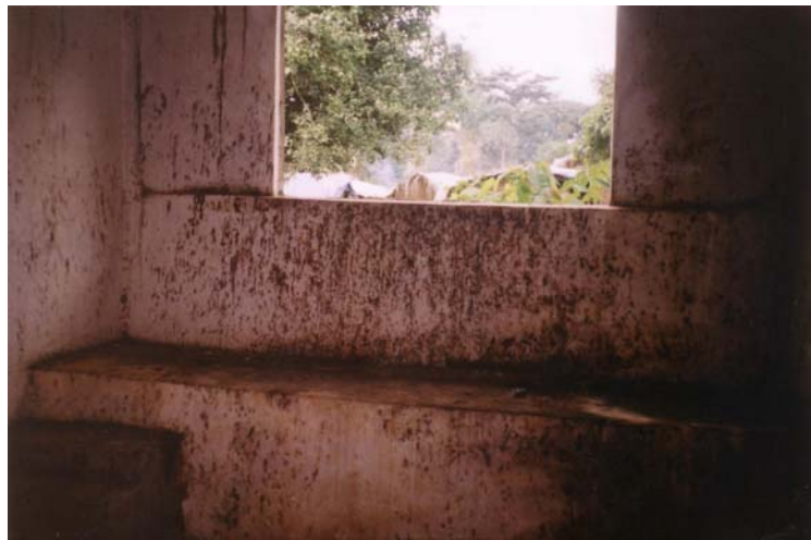
Photograph 9: The “blood stained” walls of the Slaughter House in Kailahun
