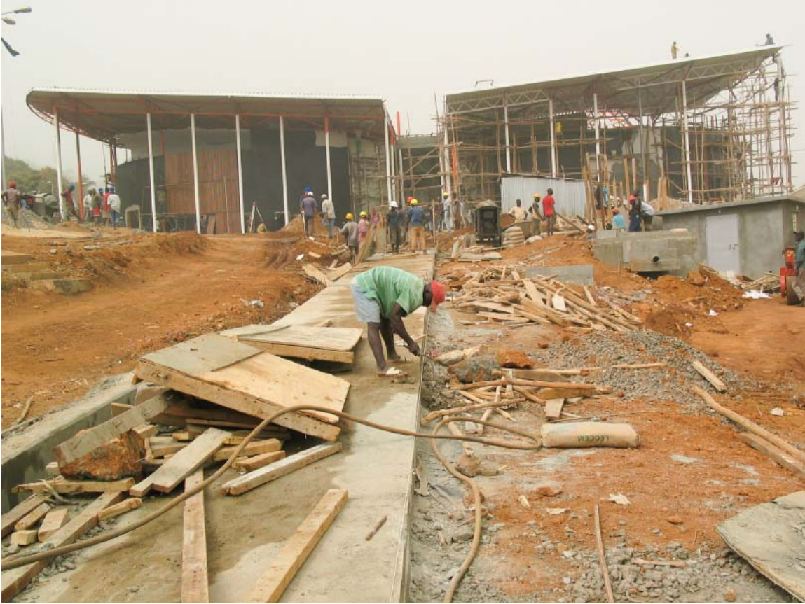
Flashback to 2004: Construction of the courthouse.
