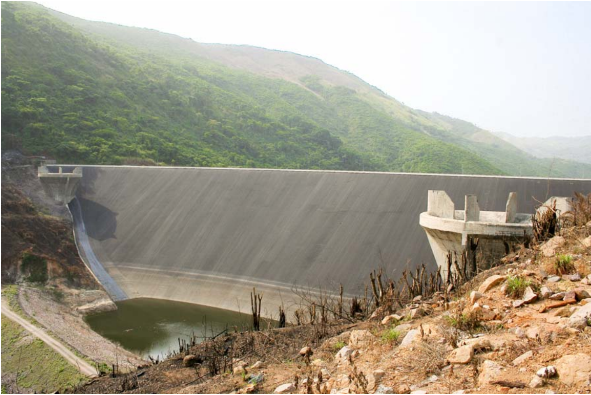
The dam at the Bumbuna Hydroelectric Project
