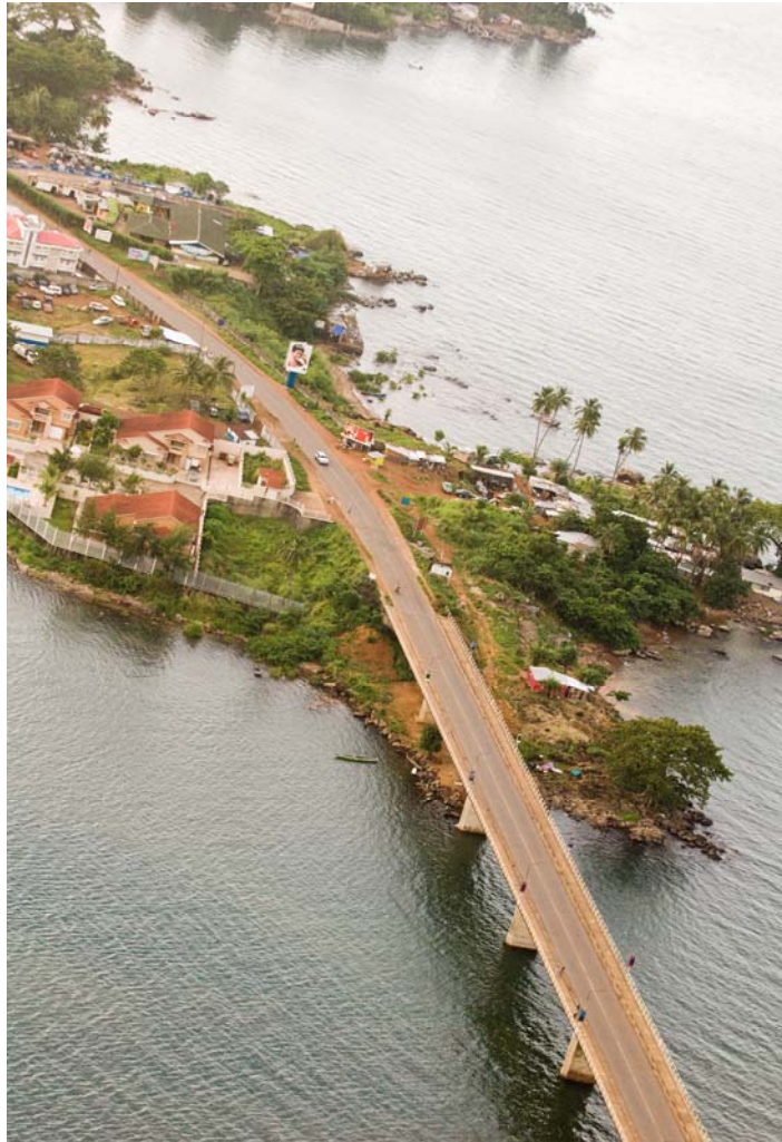
An aerial view of the Aberdeen Bridge
