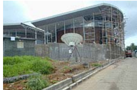
The court - seen here while still under construction
