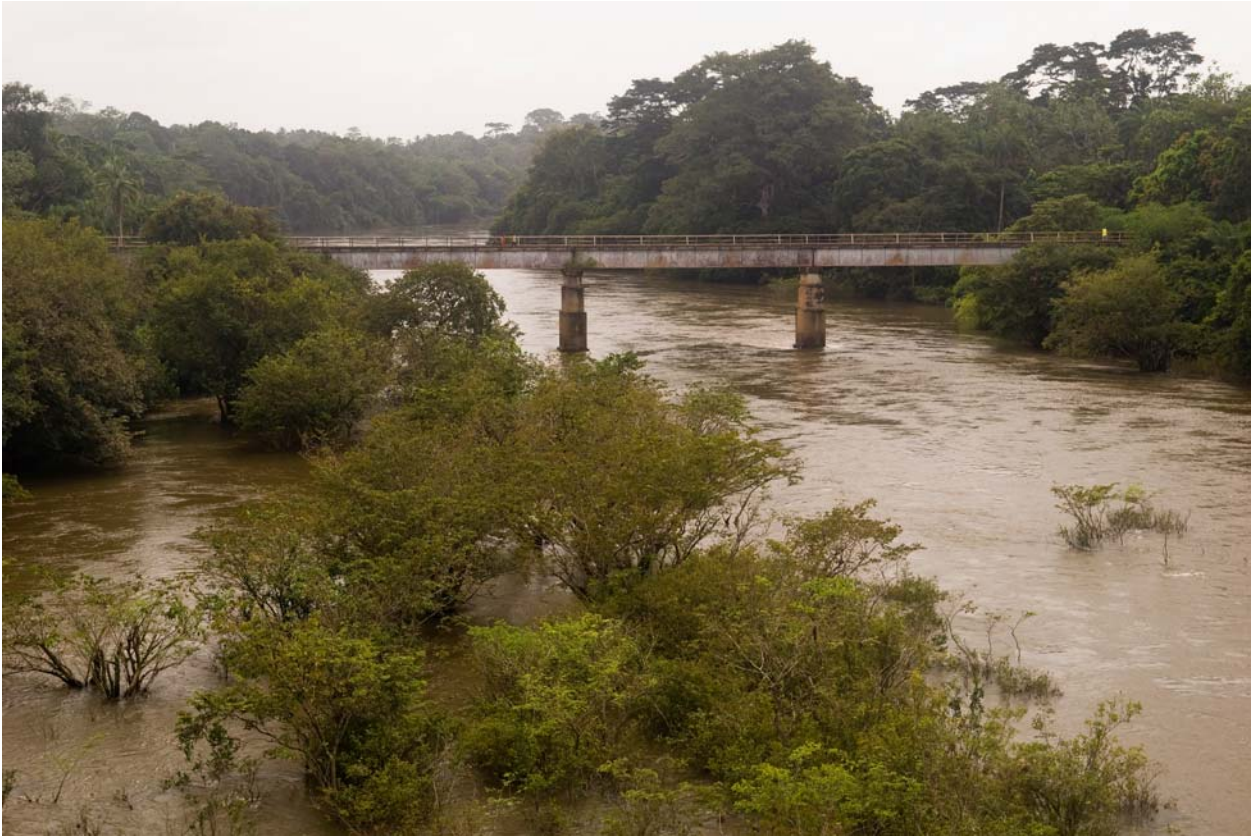
The River Rokel bridge at Magburaka
