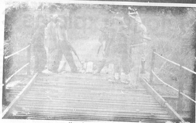
Kamajos securing a bridge
