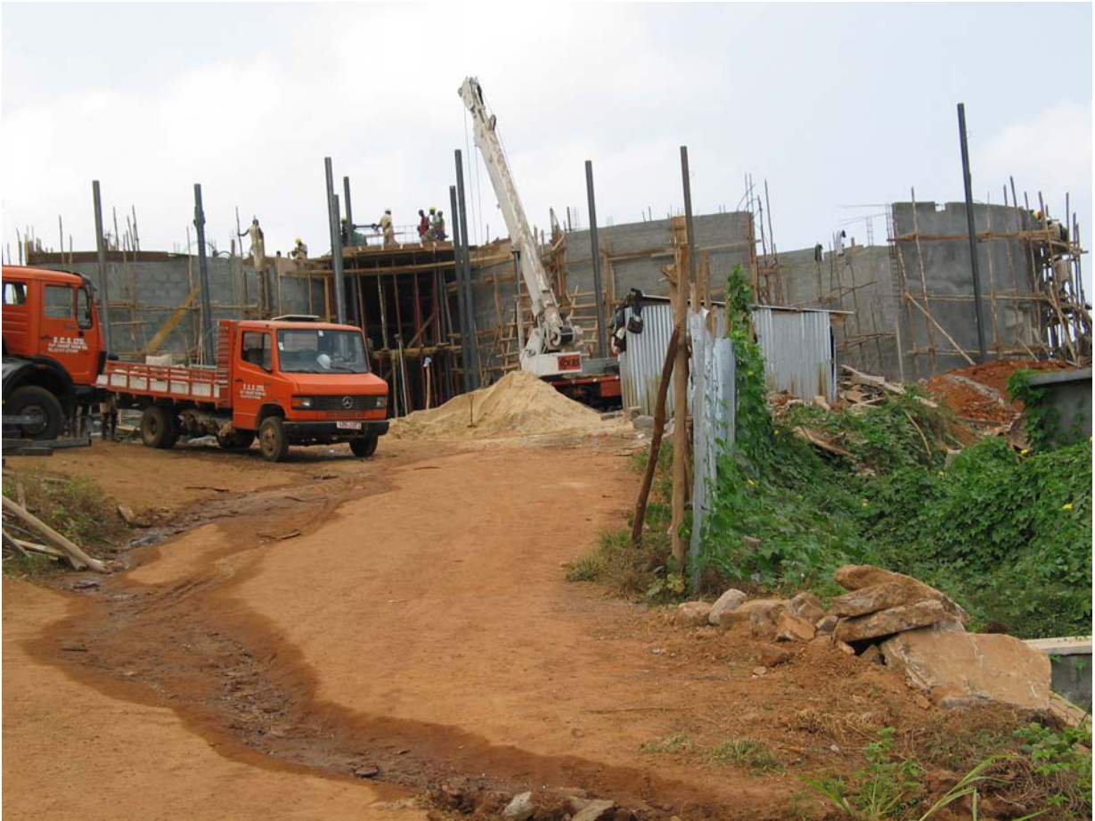
Flashback to January 2004: Construction of the SCSL courthouse
