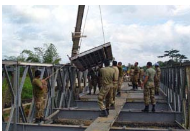
UNMIL Pakistani military engineers at work on the bridge
