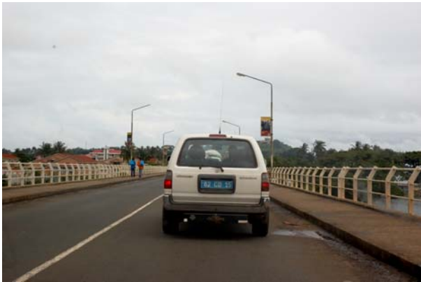
...and over the Aberdeen Bridge.
