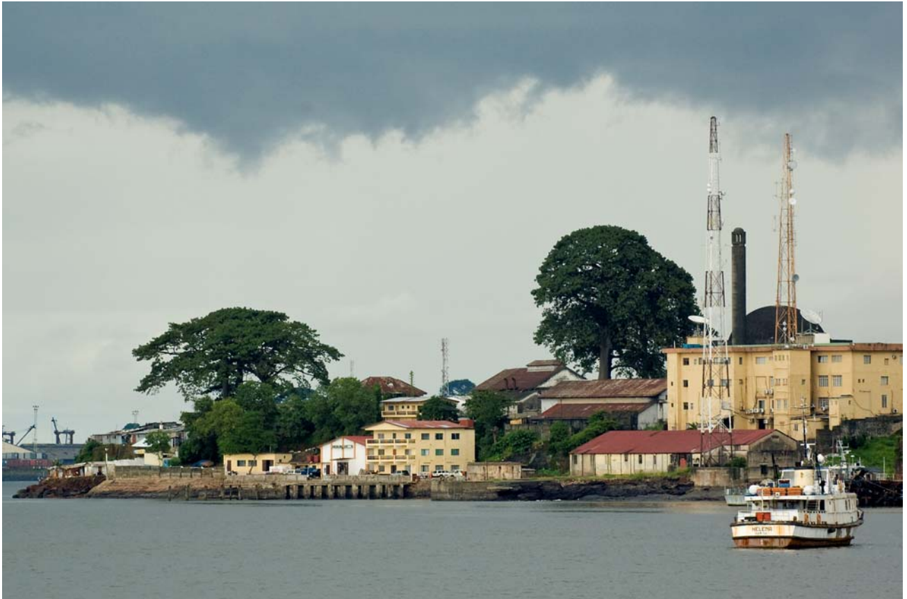
A rear view of SIERRATEL headquarters in downtown Freetown with its tall masts.
